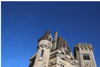
16 – Tour carrée, Villa Mors
